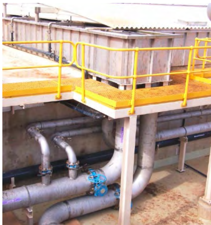
The multi-nozzle discharge of the MMS SideFeed™ settler allows neat piping in a head to head layout
